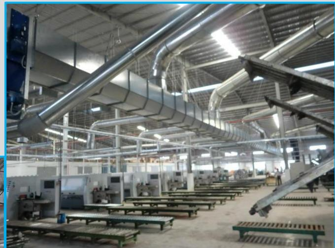
AireWorks Solutions Multiflow channel is a vacuum manifold, which ensures constant suction from all machines at all times. Pressure in the channel is kept constant by speed-controlled fans. The speed of fans is regulated automatically, to suit the required exhaust, thus reducing the energy consumption to an absolute minimum.
