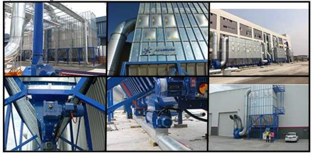
Aireworks outside baghouse collector, baghouse houses with fan and required sq/ft of filter media 7:1 air to cloth ration required for efficient filtration of fine lacquer and sanding dust.
